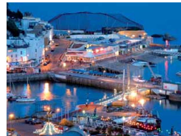
Torquay Waterfront Regeneration Project (phases 1 and 2)
